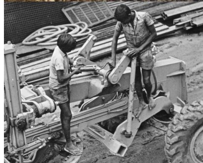
Left: The greasing crew working on the Champion road grader. This page shows examples of some of the major logging and road-building equipment brought for the project, plus Pioneer chain saws etc.
