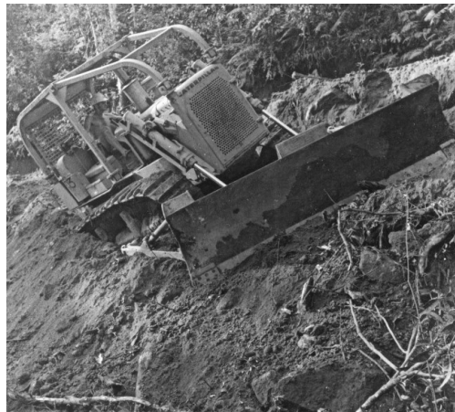
Above: Logging supervisor Jack Lewis maneuvering the D6 Caterpillar out of a difficult spot on the access road. Note the buried track.
