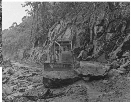
Clearing boulders from the access road with a D8 Caterpillar bulldozer after rock blasting
