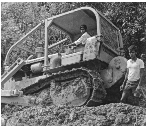
Construction of the access road. Sam is operating a D8 Caterpillar tractor. Assistant operator Dharmadasa is on the right.
