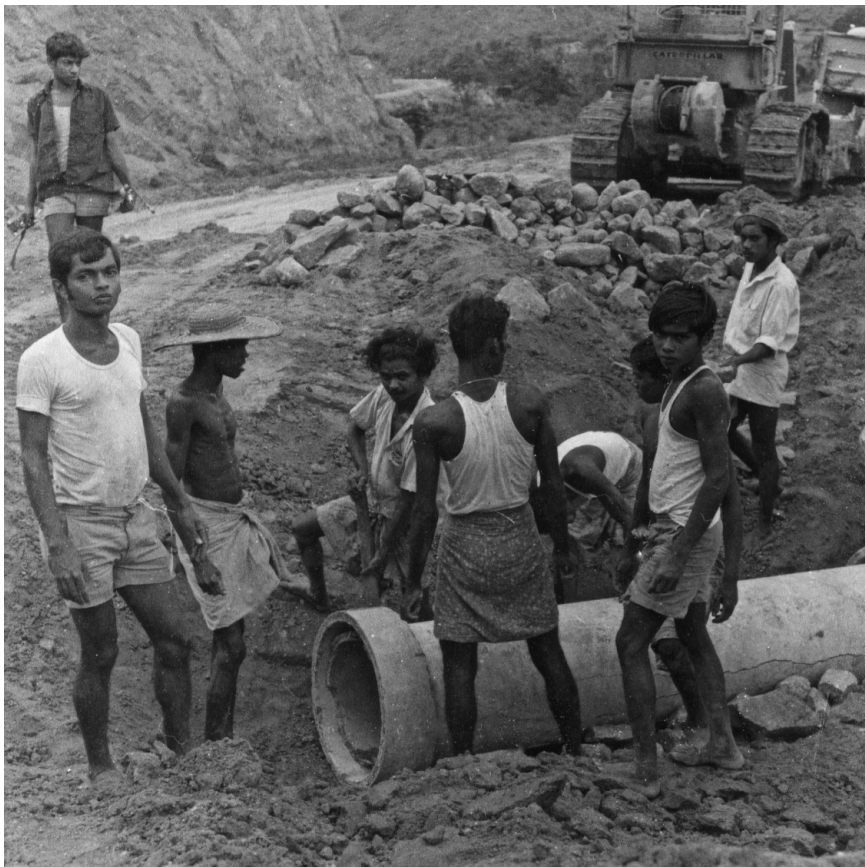
Crews laying a culverts on the access road.
